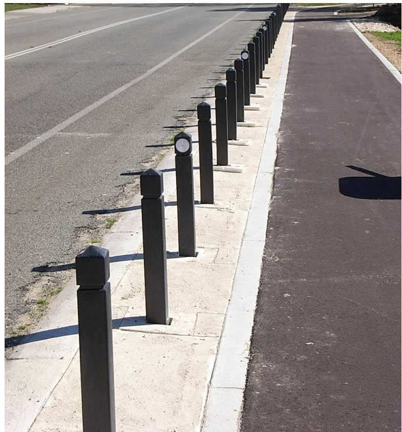
100mm bollards with reflectors
